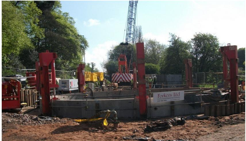
This UID project was undertaken to replace an underperforming CSO in the Compton area of Wolverhampton which, was spilling foul flow to the adjacent Smestow Brook up to 50 times annually, and was designed to intercept the existing spill pipe from the main sewer, store the first flush and then return it to the foul water system when flow conditions subside.
