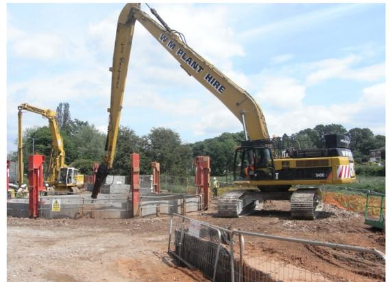
The decision was made to continue sinking the shaft as a 'wet shaft' to the full depth in order to maintain groundwater equilibrium with a base plug tremmied underwater. The standing water level in the shaft was 1m below ground level.
